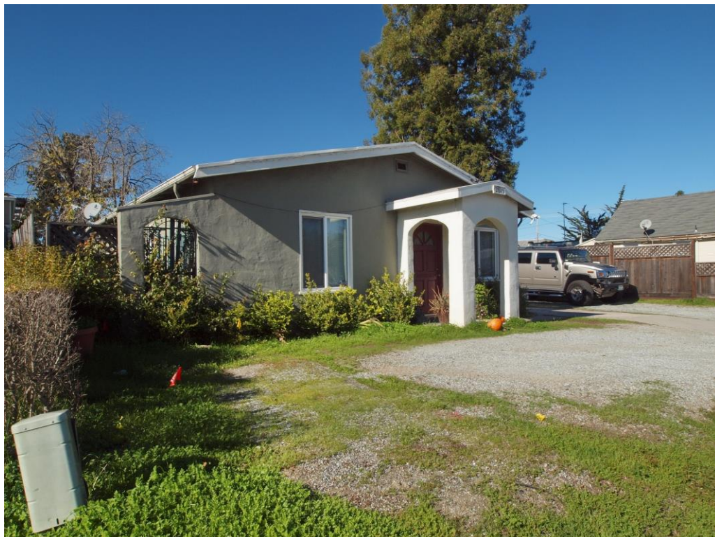
Front facade, viewed facing northwest.
