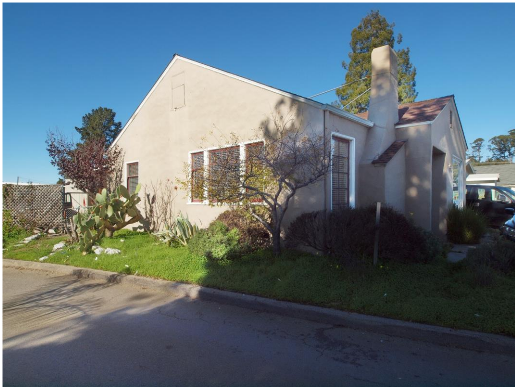
Side elevation at car wash, viewed facing northwest.
