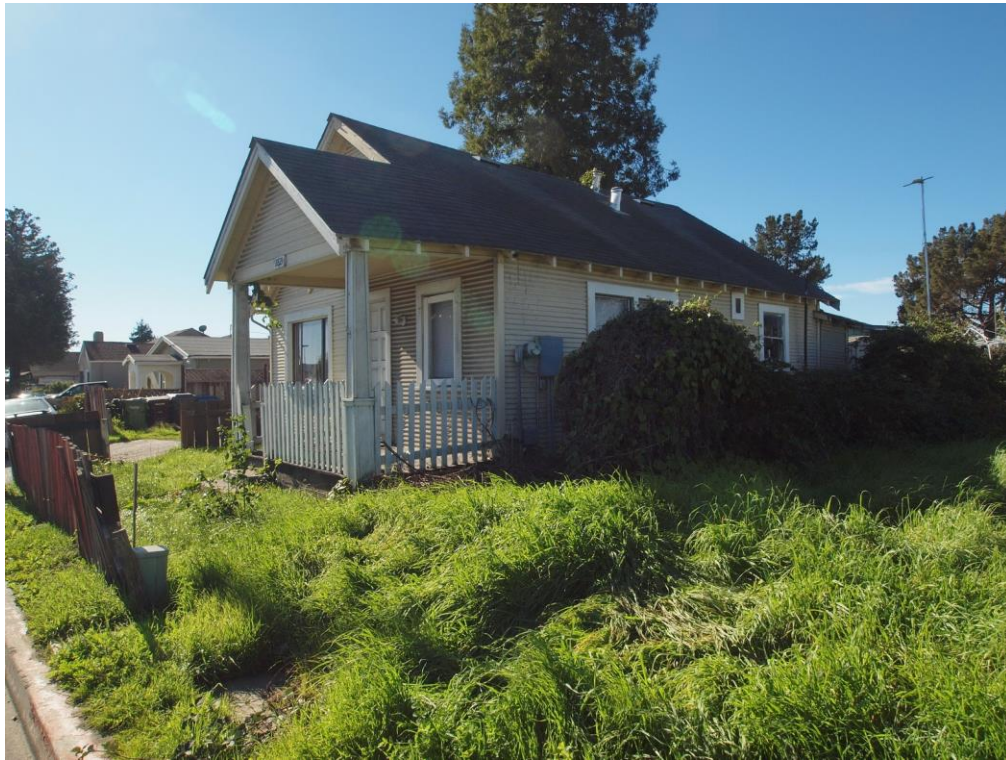
At driveway entry, viewed facing northeast.
