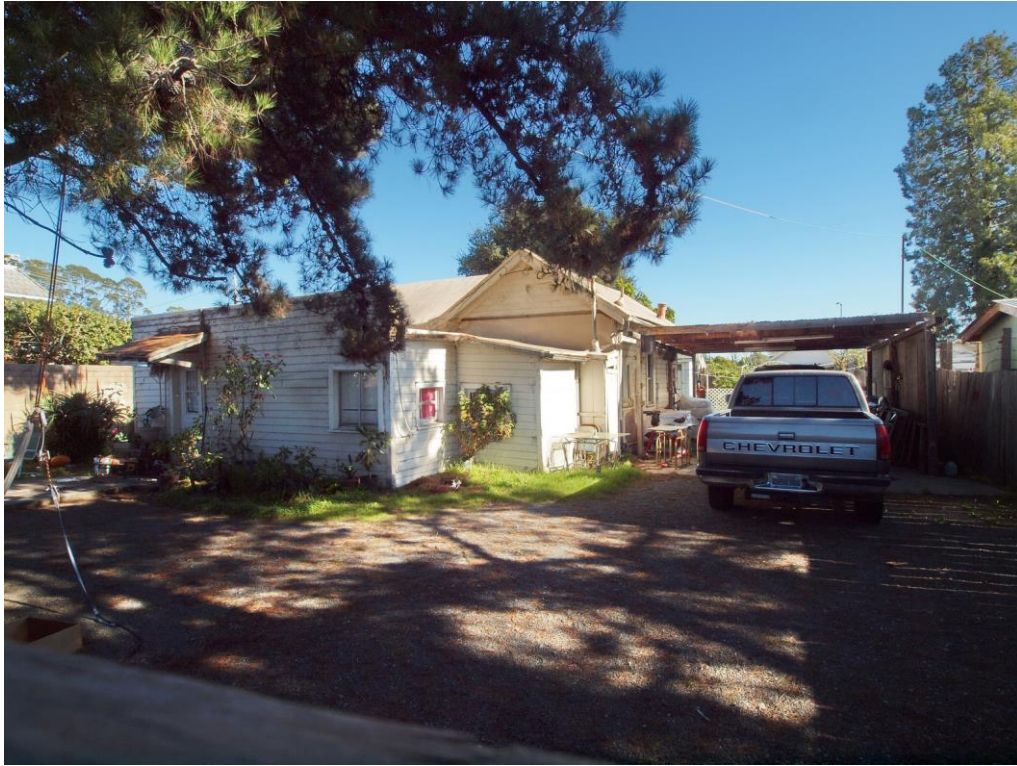
At driveway entry, viewed facing northeast.
