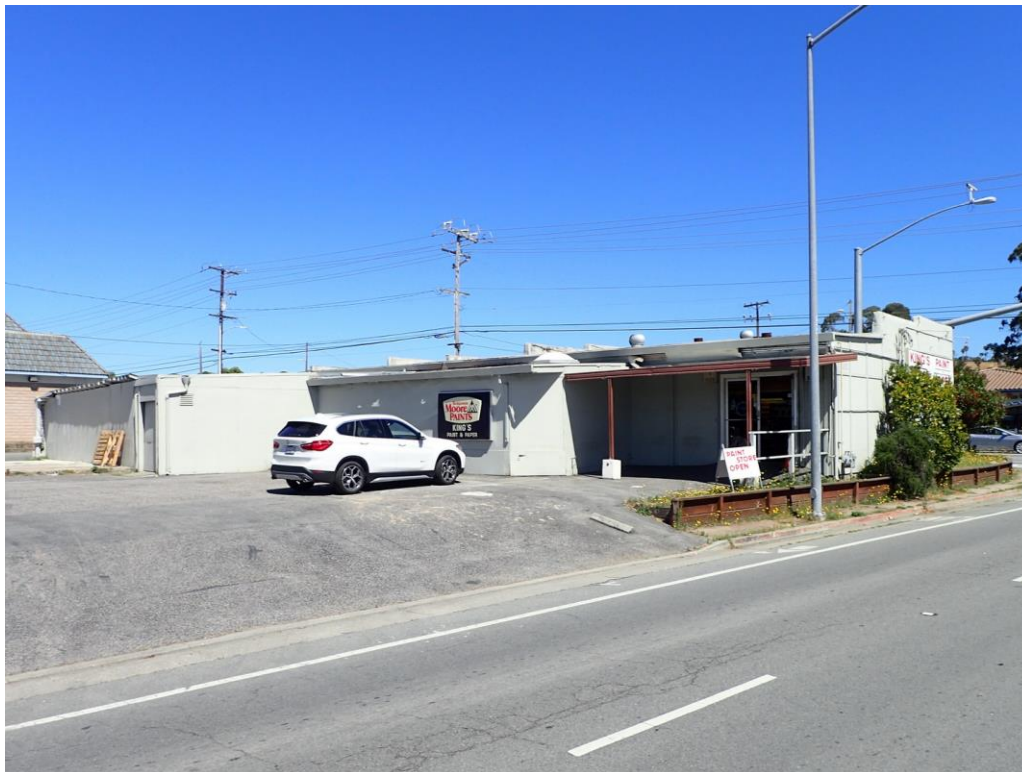
Rear entry and additions from 41st Avenue, viewed facing northeast.
