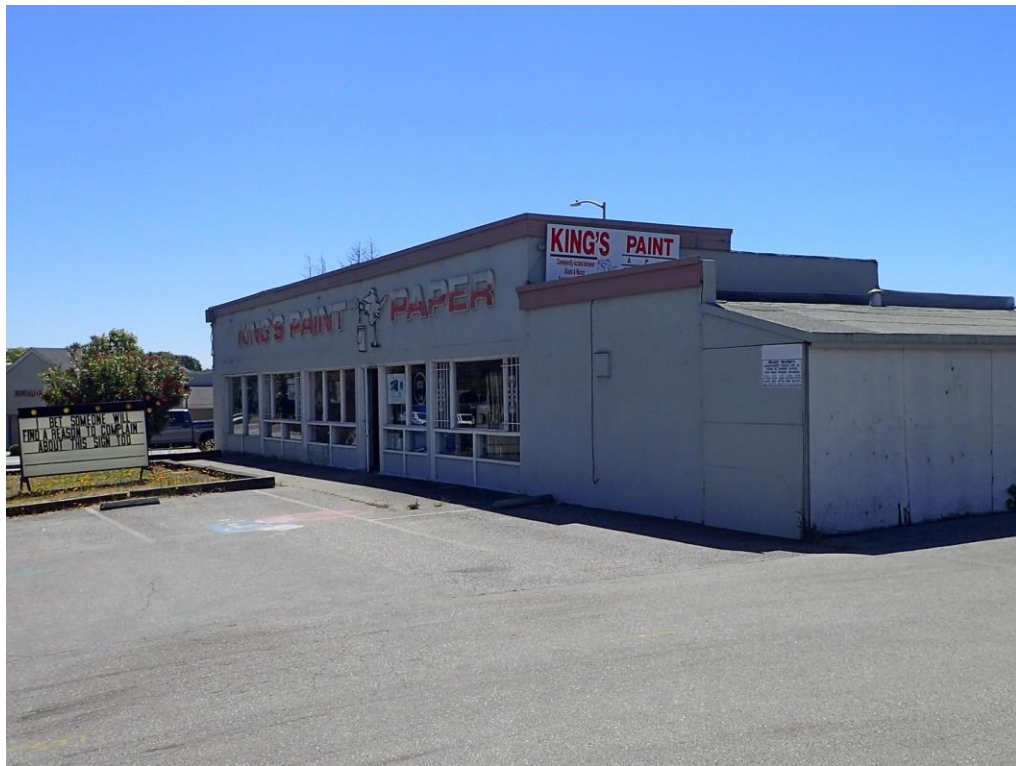
View of front façade facing southeast.
