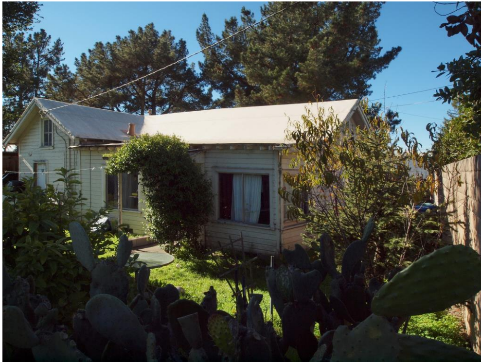
East side of house, viewed facing southwest.
